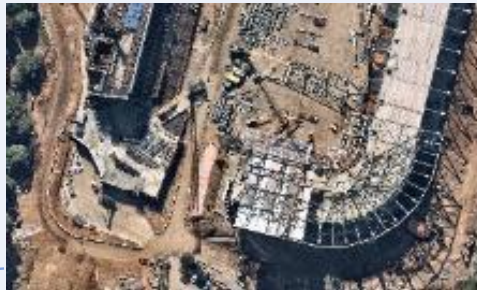
CRITICAL INFRASTRUCTURE MONITORING
